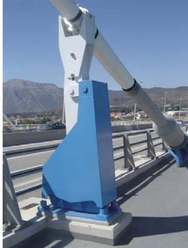
Fig. 6 Cable stays external hydraulic dampers
